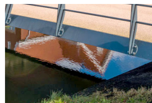
Thorca Bridge dek
